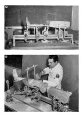
Fig. 3. Alignment duplication jig. A, Adjustable leg mounted in jig. B, Adjustable leg has been removed and wooden set-up substituted. Prosthetist is sawing shank to proper length.
