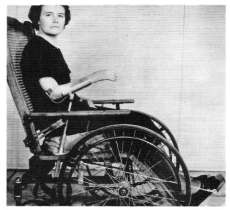
Fig. 1. "An ingenious device" supplied in 1936 to a patient at Georgia Warm Springs Foundation; also known as a "foot-operated feeder "
